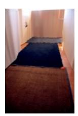
floors. It is important to consider sizes of carpets when laying them; in large areas, placing carpets of the same dimensions beside each other creates less overlap and is thus more efficient. When laying carpets it is important to avoid gaps but again, keep overlap to a minimum.
