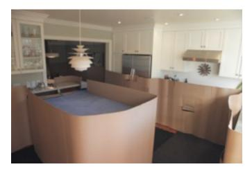
Walls are generally protected with cardboard that comes in rolls 4' wide. Cardboard is generally taped to the wall with masking tape, but in situations where surfaces are extra sensitive, creative cutting and wrapping can allow the cardboard to be supported by taping to itself or by making cardboard "tab and slot" fastenings.
