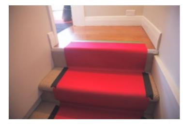
Neoprene stair runners may be taped to stairs to protect carpet, wood or stone. When applying stair protection,
